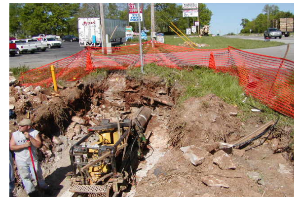
Installation of new water mains along Morgantown Road.
